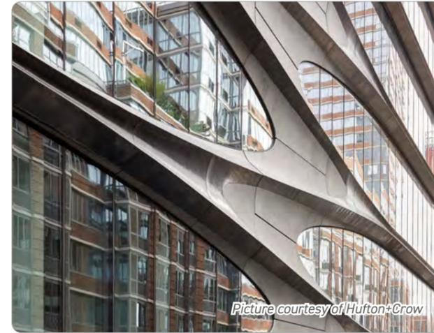
Type 304 (UNS 30400) stainless steel features a blackened finish achieved by an antiquing process, light orbital brushing and hand tinting. The panels were engineered, cut, welded and installed by Philadelphia-based fabrication group, M. Cohen and Sons. Over 350,000 man hours were invested to produce these and bring the architect's vision to life.
