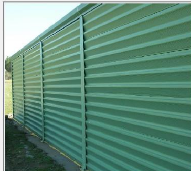
Ferritic sound absorbing panel (prototype), Rome (2007).
