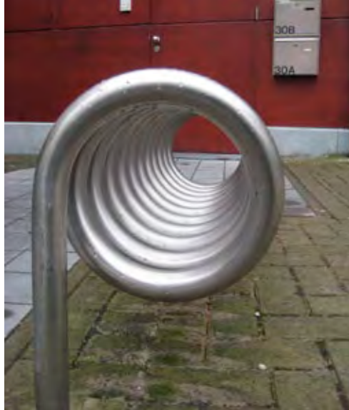
Cycle racks made from spiralling tube combine ease of installation, mechanical strength and visual attractiveness.
