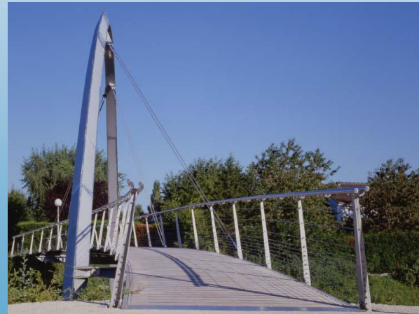
Charvaux Footbridge, Andrésey, France, Single-arch suspended footbridge in 316 (1.4401) stainless steel
