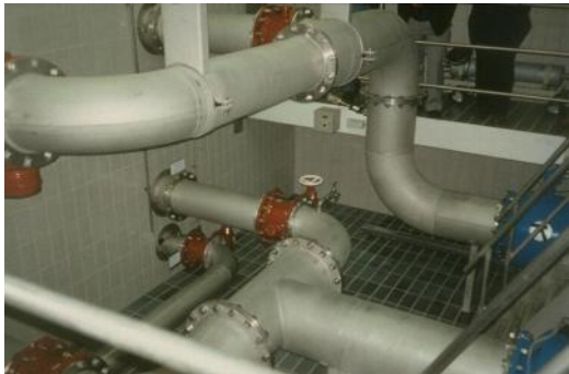
Potable water treatment
