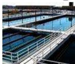
Potable water plants ②
